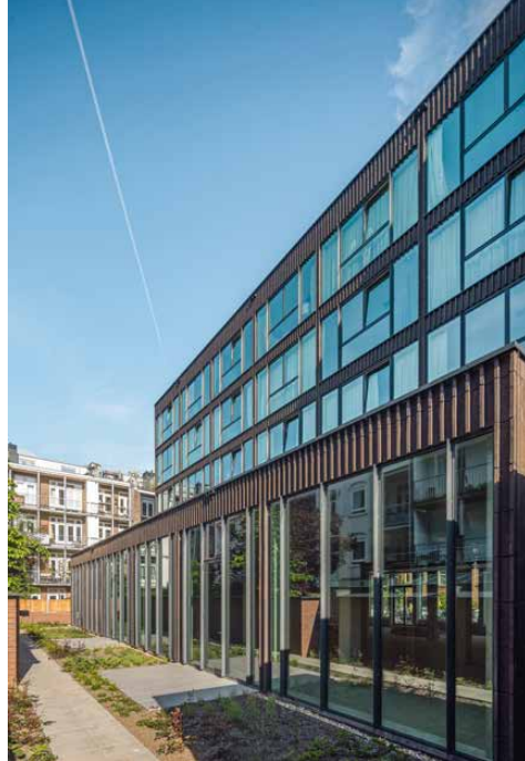
The protruding ground floor façade facing out onto the courtyard is also brick clad.
